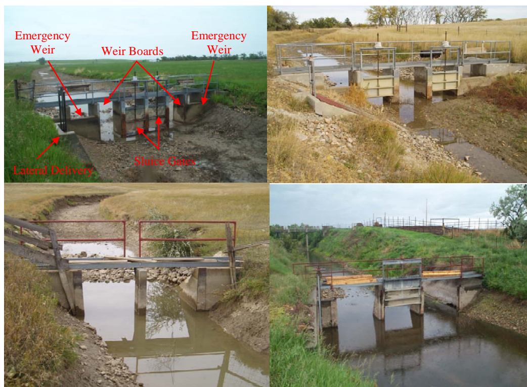
Figure 3-7. Four Examples of Check Structures Along the South Canal, Belle Fourche Irrigation District. Each has a Different Combination of Weir Boards and Sluice Gates With the Exception of the Bottom Left Which has no Sluice Gates. Each Structure has, in Turn, a Unique Rating Curve.
