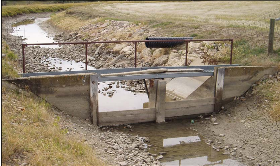
Figure 4. A common Reach 4 check structure.
