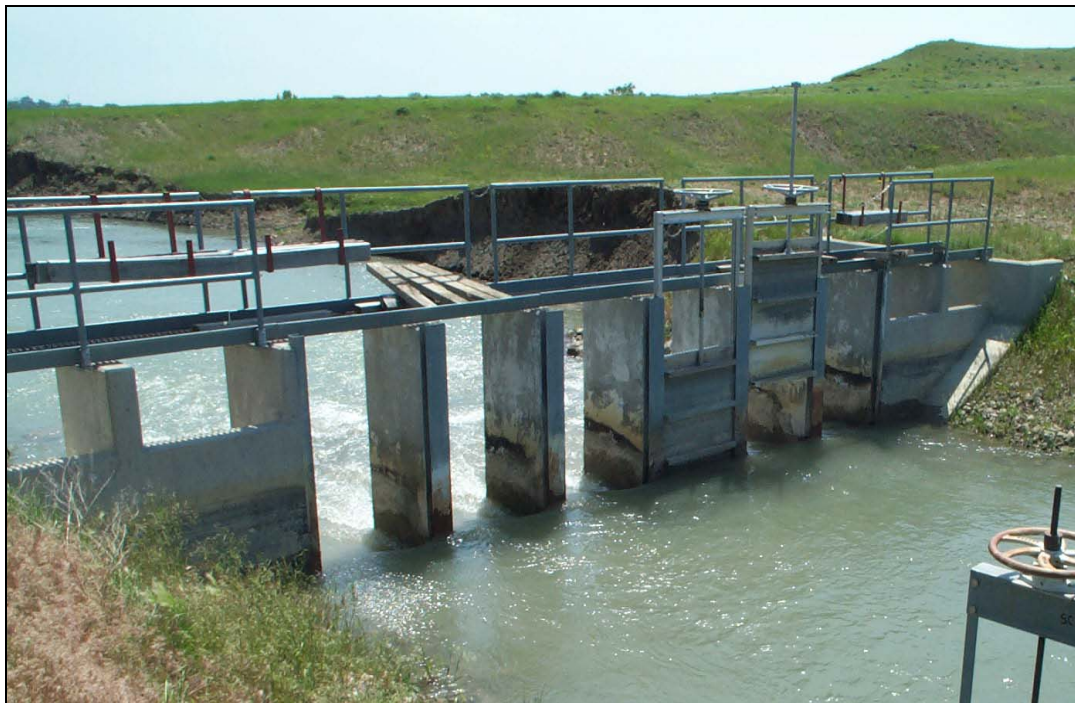
Figure 5. Meyer Check structure on Reach 1.
