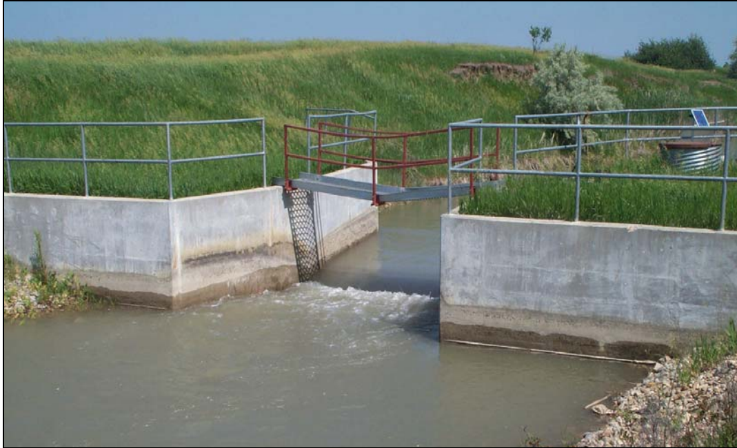
Figure 10. Belle Fourche River Siphon Flume outlet.
