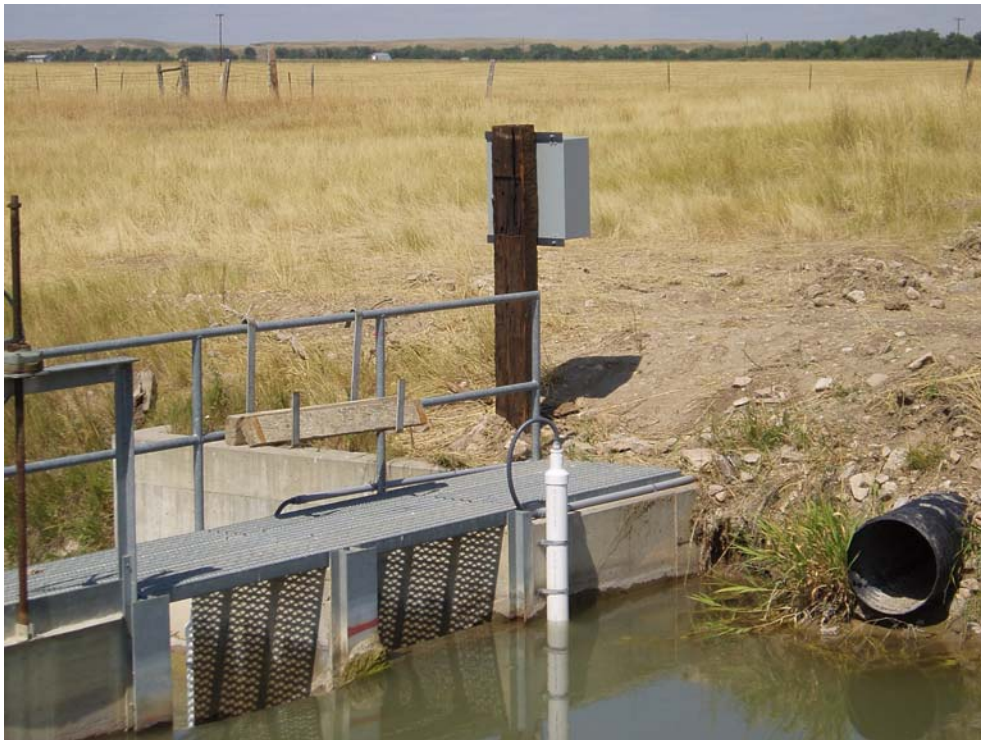
Figure 3-1. Gate Automation Unit Installed in the Belle Fourche Irrigation District.
