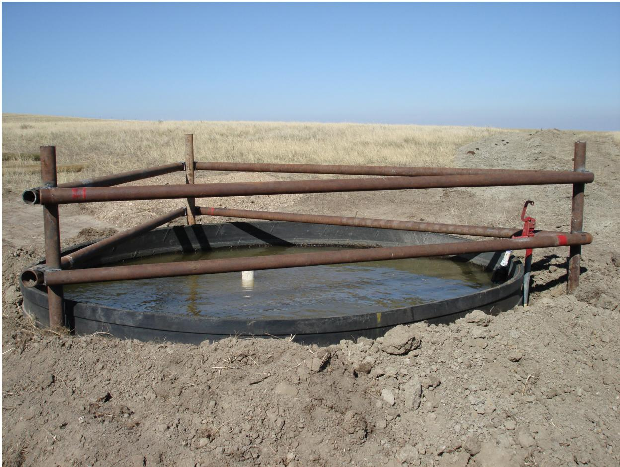
Figure 3. Example of off-stream livestock watering tank implemented with Segment III implementation funds.
